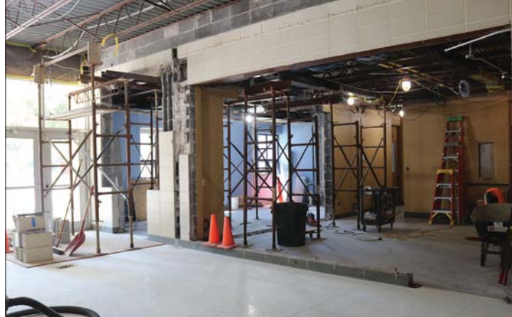
Above: Current construction on McDonell Central Catholic High School main entrance with the front wall of the school office and the wall between the school office and campus ministry room removed.
