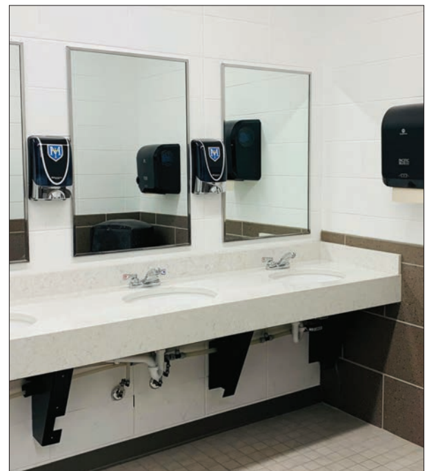
Updated women's bathroom in the commons at McDonell Central Catholic High School and Notre Dame Middle School. The bathrooms previously were outfitted with the original fixtures installed in 1965.
